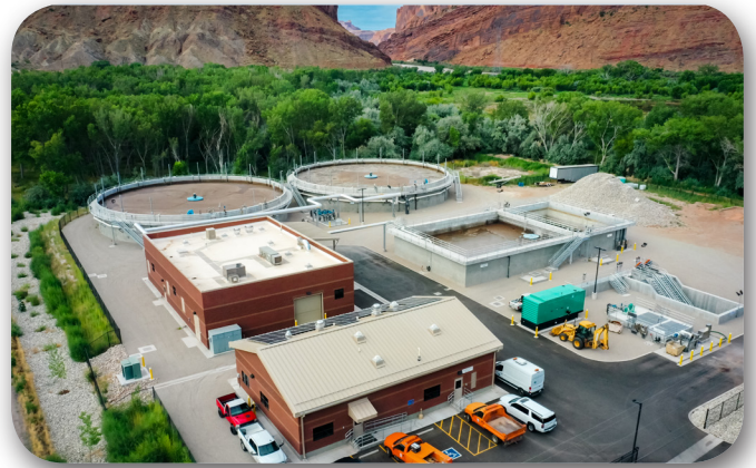
AquaSBR® System at Moab Water Reclamation Facility - Moab, UT
