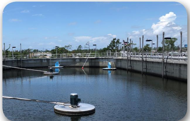
This 3-basin AquaSBR® system was built to expand the capacity of the existing oxidation plant which was re-purposed for storage tanks. The system has been designed to easily add a fourth SBR basin to increase treatment capacity in the future. The SBR system started operation late 2019.
