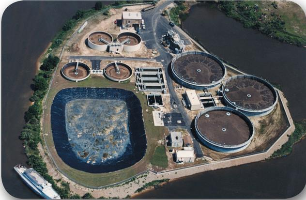
The AquaSBR® system at Millville is a 3-basin system designed to meet advanced wastewater treatment standards. The plant has been in operation since November of 2000 and has provided the Panama City area with a low cost, efficient system that consistently meets its treatment objectives.
