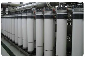
Aqua MultiBore® Polymeric Membrane Installation
