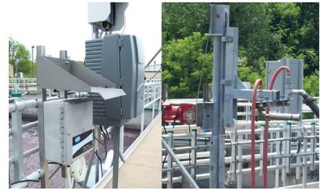
The IntelliPro system is a PC based process control system that receives, interprets and proactively responds to the loading variation in the biological process.
