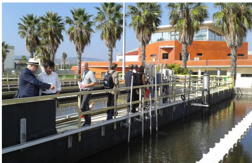
Figure 11: Full Scale Installation Frielas, Portugal
