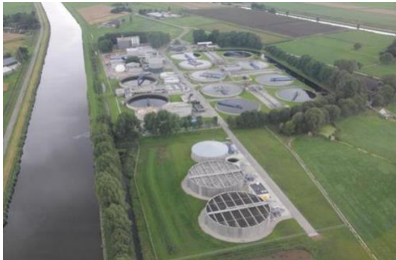
Figure 10: Full Scale Installation Gammerwolde, NL
