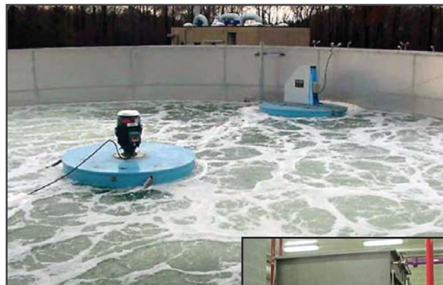
York River's AquaSBR ® basin in operation (top) and 4-disk AquaDisk ® filter located inside a small building (right).
