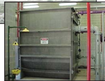
York River's AquaSBR ® basin in operation (top) and 4-disk AquaDisk ® filter located inside a small building (right).
