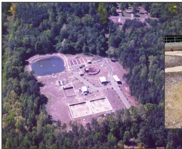
Aerial view showing the 2-basin AquaSBR ® system and a closeup of the system in operation is shown to the right.
