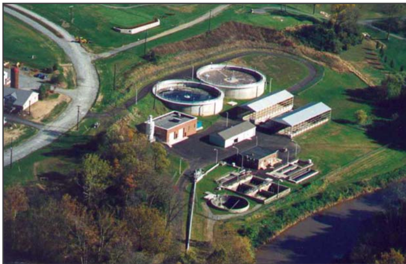
The AquaSBR ® system was constructed adjacent to the existing plant.
