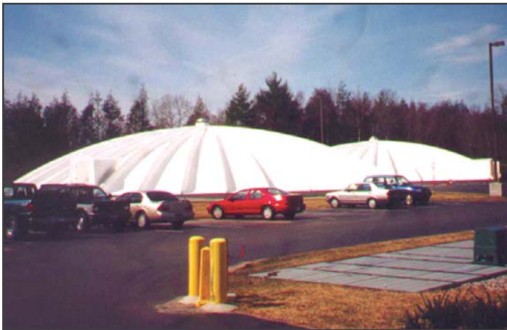
AquaSBR ® basins #1 and #2 are shown. Basin #3 is located adjacent to these two basins. All the basins have covered tanks.
