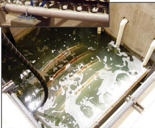
Internal view of one of the AquaDisk ® Filter units.
