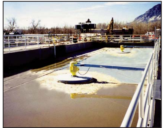
One of five anoxic basins utilizing AquaDDM ® mixers with a pivotal mooring arm.
