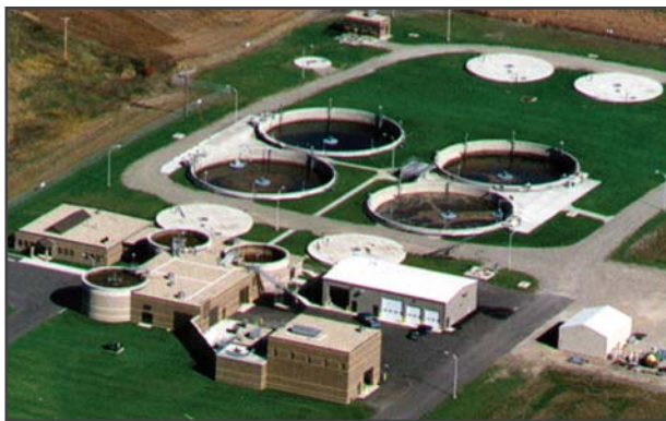
Aerial view of Clear Lake showing four AquaSBR® basins.
