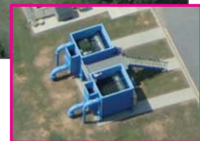
Aerial of the 2-basin AquaSBR ® system with adjacent (2) 6-disk AquaDisk ® filters.
