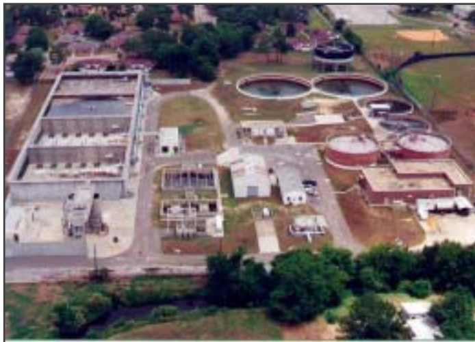
Only two of the four AquaSBR basins at KeeganBayou are currently needed for operation.
