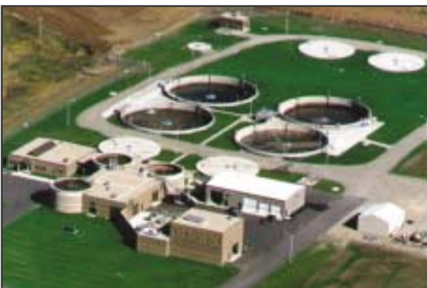
Aerial view of Clear Lake showing four AquaSBR ® basins.
