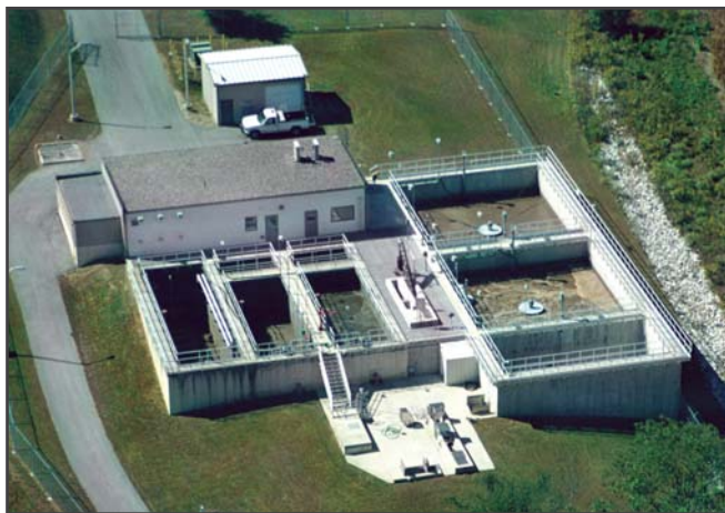
Abbottstown's dual-basin AquaSBR system is shown on the right.
