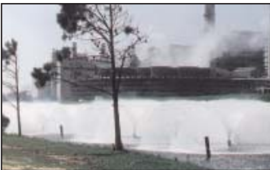
ThermoFlo units at a utility plant.
