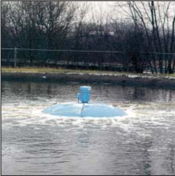
Pictured is a 15 HP Aqua-Jet II operating at an industrial facility.
