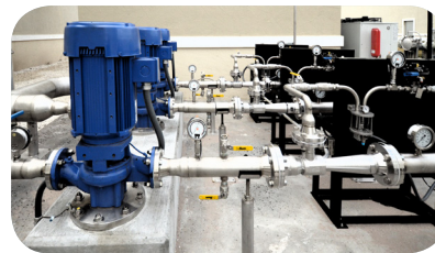
Ozone injection set detail.
