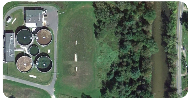
Aerial view of the 4-basin AquaSBR ® system and buildings housing the 2 AquaDisk ® filters and other treatment equipment. The plant is located nearby the receiving Housatonic River (shown right).
