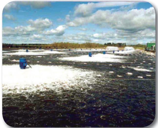
A number of MacLaren's Aqua-Jet<sup>®</sup> aerators in operation. The ThermoFlo<sup>®</sup> spray coolers can be seen in the background.
