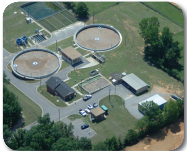
Aerial of the 2-basin AquaSBR® system with adjacent (2) 6-disk AquaDisk® filters
