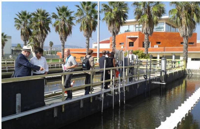
Figure 11: Full Scale Installation Frielas, Portugal
