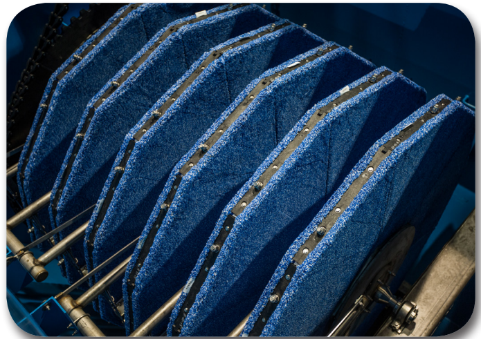
Internal view of a 6-disk AquaDisk® Cloth Media Filter
