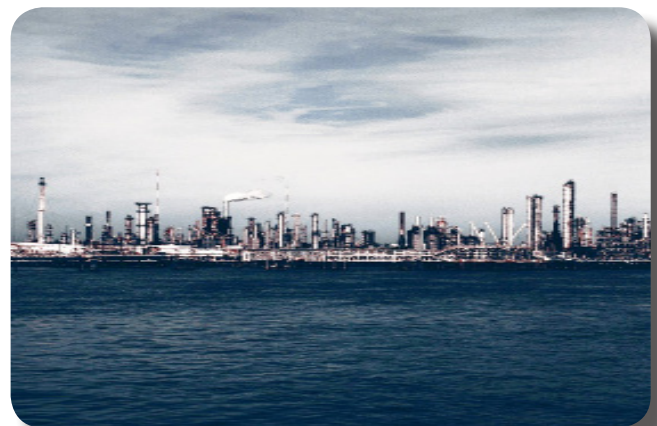
A riverfront petrochemical processing facility - Louisiana
